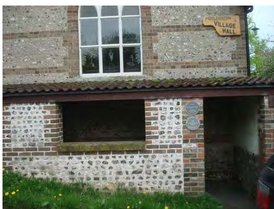
Piddlehinton Village Hall and Bus Stop
